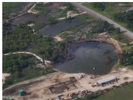
Daisetta sinkhole today
