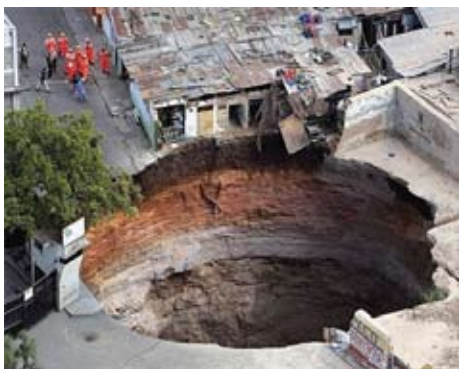
Initial Daidsetta sinkhole
